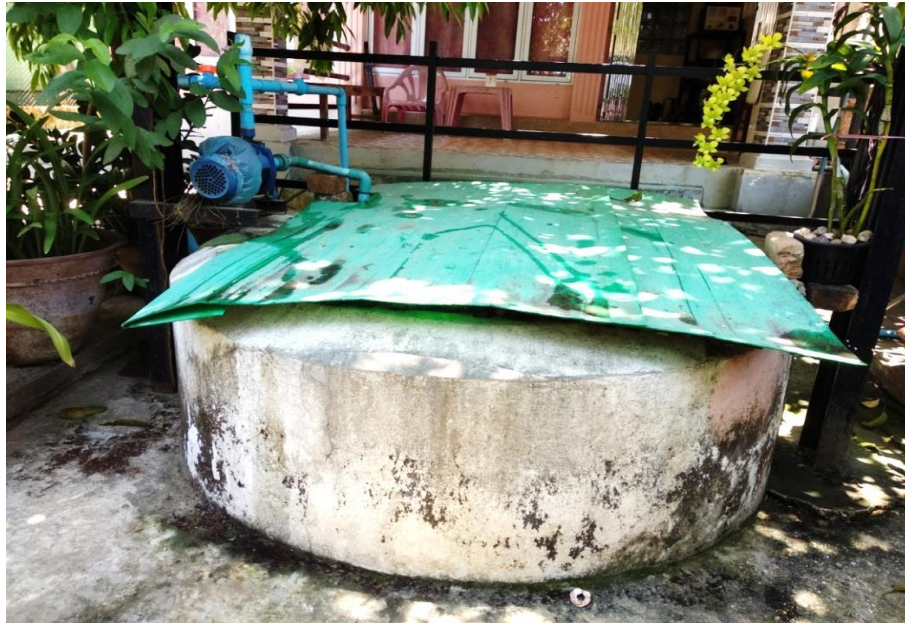
Plate 3 Surface Well of Shwegone Ward in Kyauktan Town
